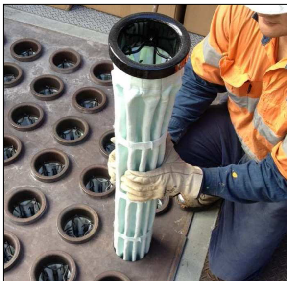
Figure 6. Installation of an extended surface filter bag (Source: Advantec International).
